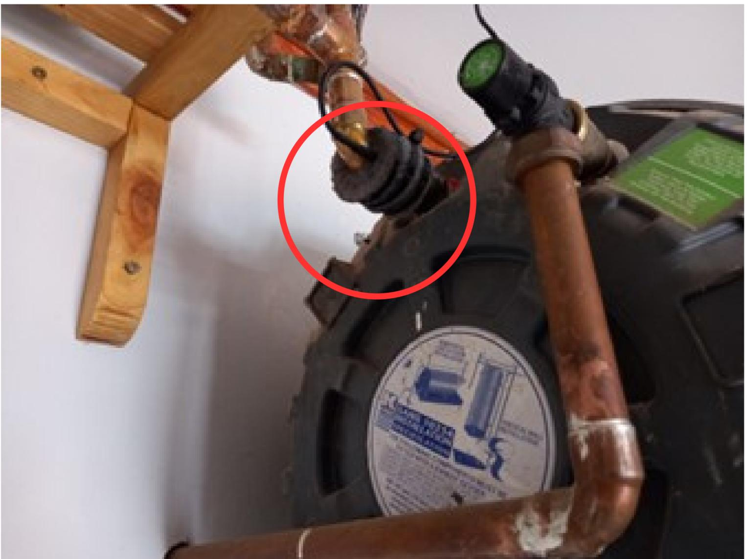
Figure 14: Temperature sensor placement
